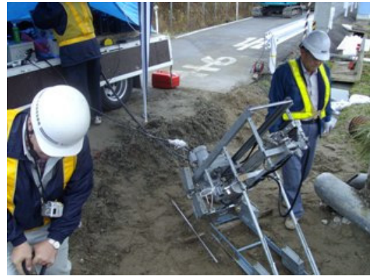
Figure 3. Appearance of slope measurement with NSW testing machine
